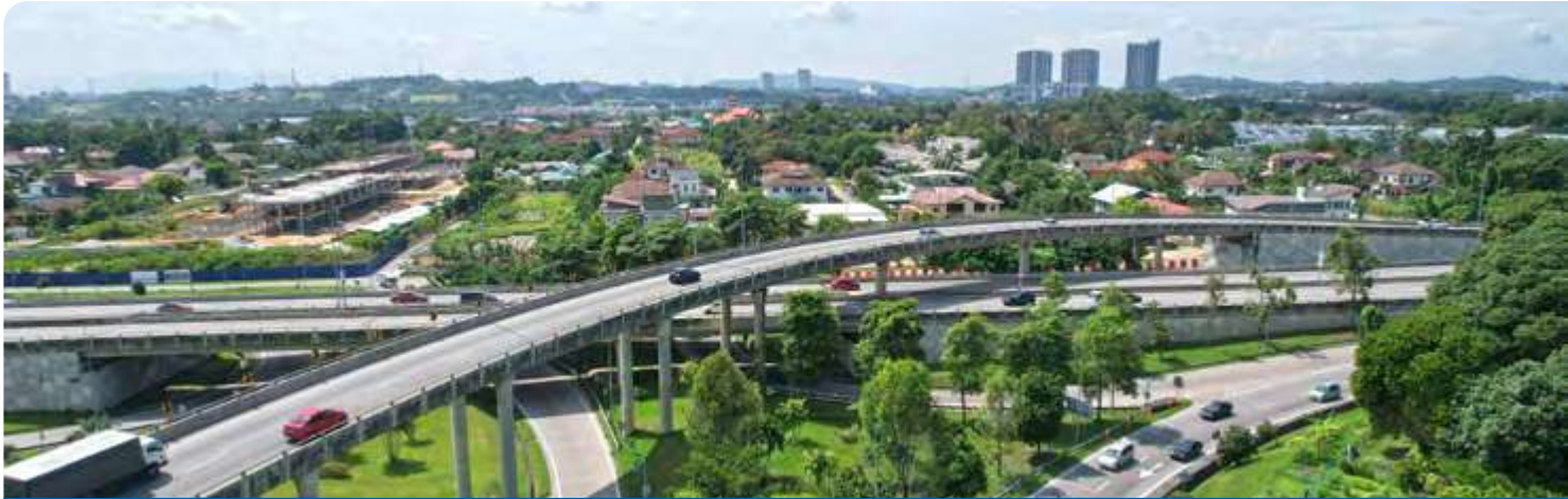
SILK - Delivering efficient, high-capacity connectivity across the Klang Valley.
